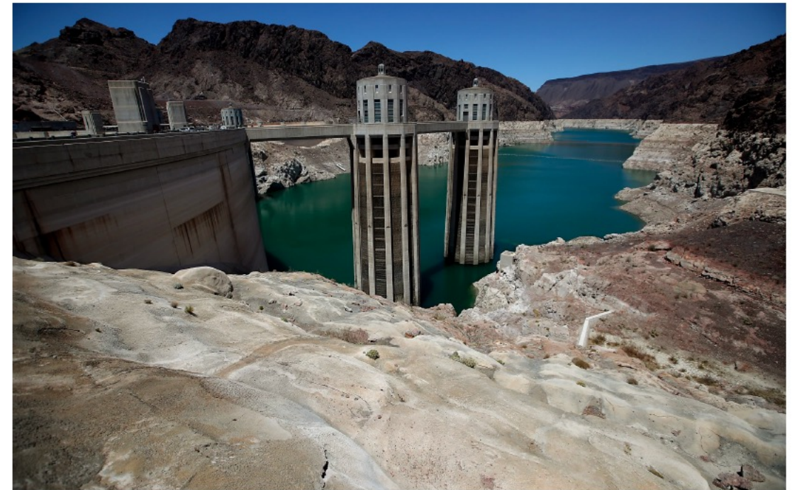
The intake towers that feed Hoover Dam's power generators are almost fully exposed as the Lake Mead water level continues to decline. (Luis Sinco/Los Angeles Times)
